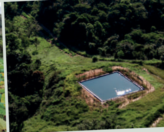
A 470,000-liter reservoir ensures irrigation. This is a very important factor, as the soil here is sandy.
