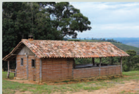
RANCHO DO AREIÃO – This ranch in adobe, wood and no plastering was rehabbed and updated to enhance the landscape. Currently, it is used for open-air meals.
