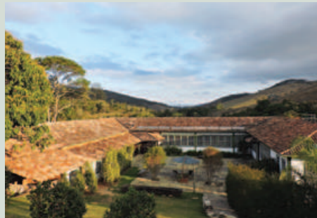
POUSADA (Lodge) – The house was erected in 2008 from mainly recycled demolition materials (mostly taken from the surrounding area). Traditional building techniques were employed. The veranda was inspired in the former main house of Fazenda do Engenho.
