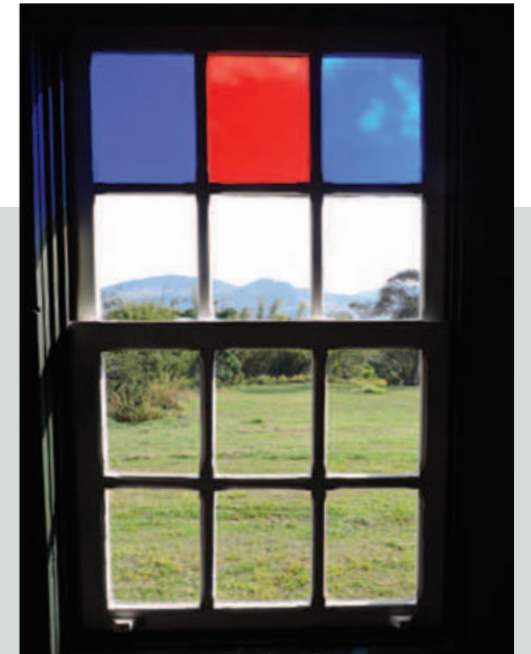
The colored glass windows seen in many buildings at Reserva are a poetic touch to the landscape
