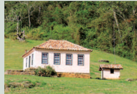
CASA DO BENJAMIN – Just like Casa do Zico, this house had the exterior appearance preserved while the interior was modified to enlarge its tiny rooms. The house painting is soil-based: naturally pigmented material called oca.
