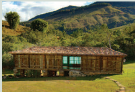
SPA – This construction used to be the farm's barn. It was demolished and rebuilt with the same material (stone and wood) and transformed into a therapies center.
