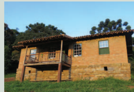
CASA DO LUNA – Built in 2016, this house features a hybrid technique. It mixes stone and recycled oversized bricks. It is located at the entrance of Mata do Luna and serves as lodging for visiting researchers.
